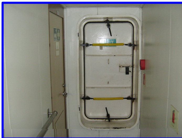
Watertight door effectively secured
