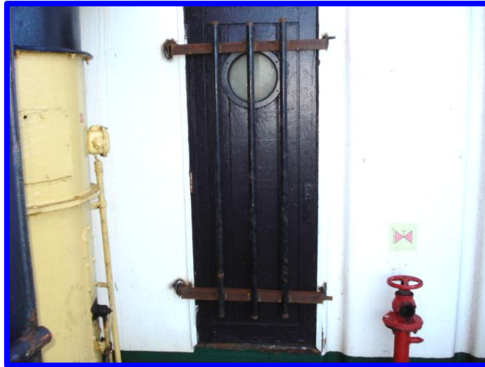
Extra strengthening on at risk doors before the citadel
